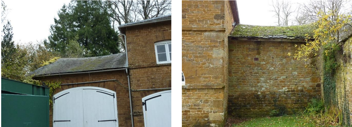
Roof slopes P (left) and Q (right)
