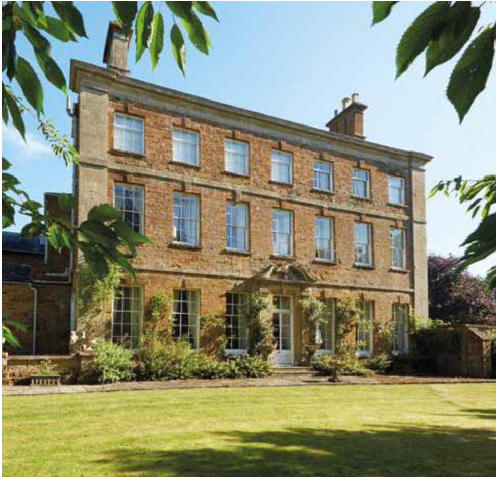
South elevation showing use of light-coloured Cotswold stone as an architectural design feature. The same stone is used in the barrels of the SW and NE chimneys.
