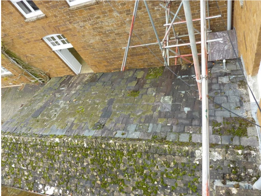
Roof slope G
