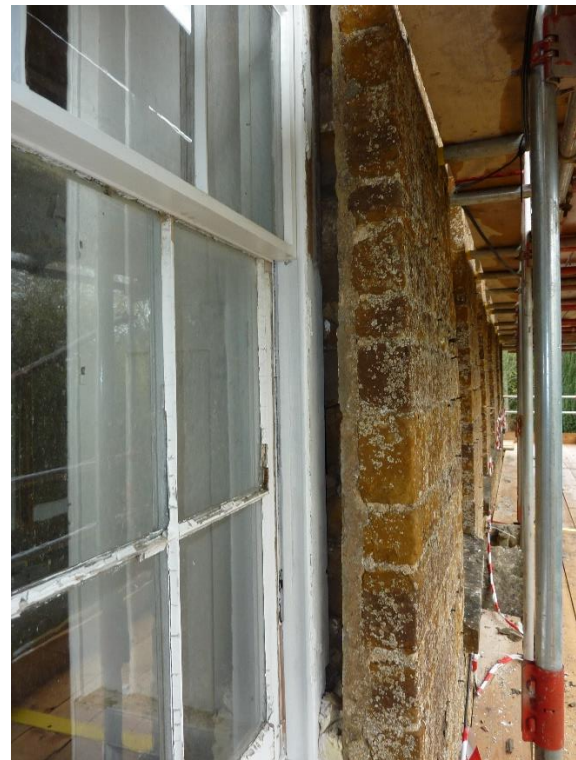
Cracked and failed cement fillets between south sash windows and facing ashlar stonework
