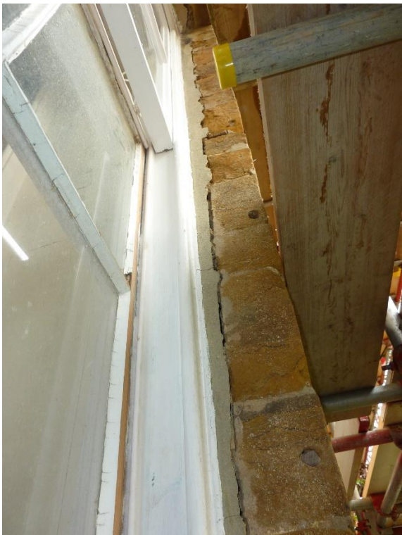
Cracked and failed cement fillets between south sash windows and facing ashlar stonework
